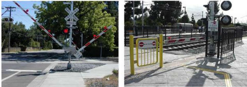
**Figure 6: Pedestrian Automatic Gate Examples**
