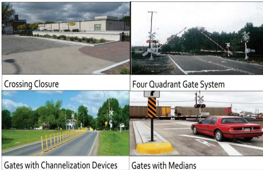
**Figure 2: Examples of Supplemental Safety Measures for Quiet Zones**
