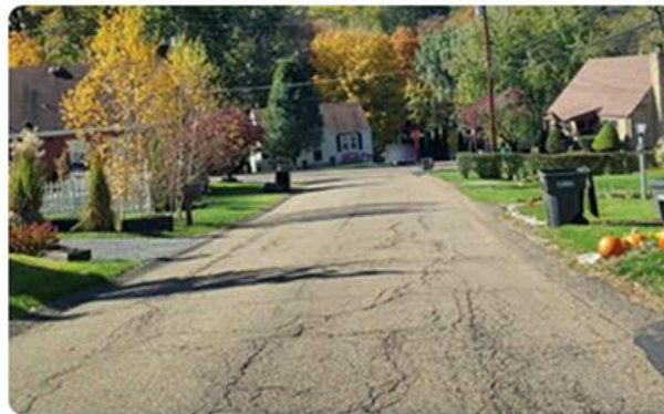
Fatigue Cracking
