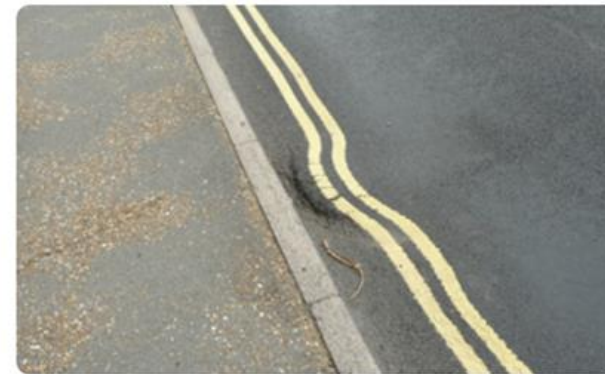
Pavement Distortions
