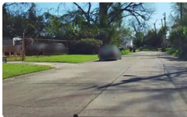
Transverse/Longitudinal Cracking
